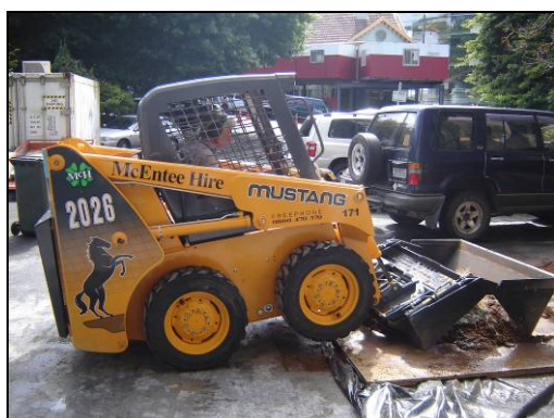
Figure 6: Compact Loader mixing soil
